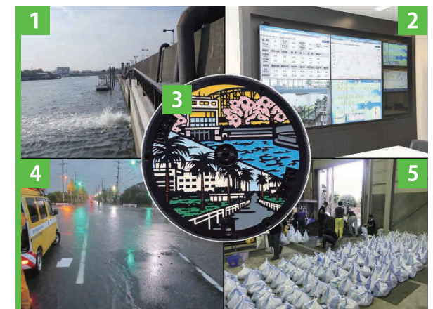
① Pumping stormwater into the river through a drainage pump station outlet ② Centralized control system screen in the disaster response headquarters displaying river and weather information ③ Urayasu City's design manhole cover ④ Staff dispatched with a maintenance vehicle due to road flooding ⑤ Preparing sandbags at a pump station in anticipation of levee breaches during Typhoon Source: Urayasu City
